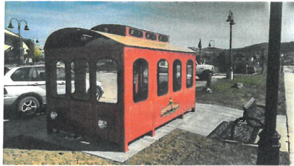
Figure 12: Cripple Creek Bus Shelters
